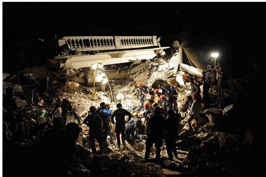
PORT-AU-PRINCE, Haiti (Jan. 17, 2010) Members of the Los Angeles County Fire Department Search and Rescue Team clear debris at a collapsed building in downtown Port-au-Prince. (U.S. Navy photo by Mass Communication Specialist 2nd Class Justin Stumberg/Released)
